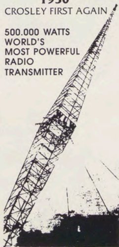
WLW's Tower at Mason, Ohio
