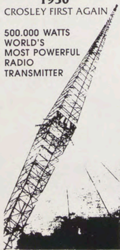
WLW's Tower at Mason, Ohio
