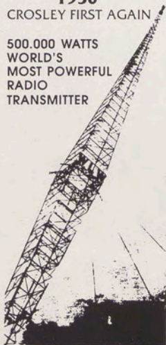
WLW's Tower at Mason, Ohio
